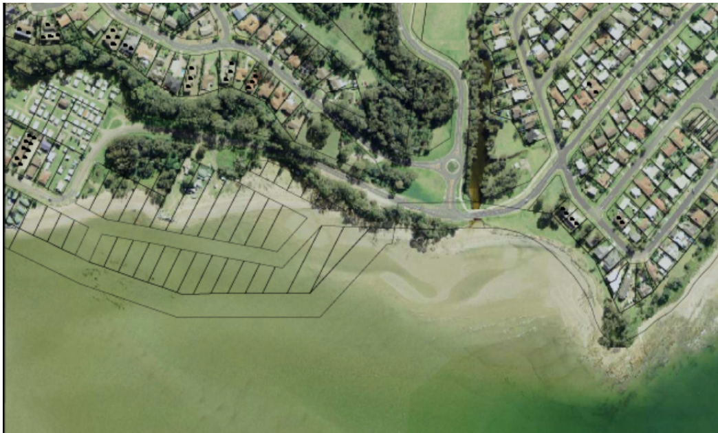
Shoreline recession at a coastal erosion hotspot, courtesy of Eurobodalla Shire Council.
